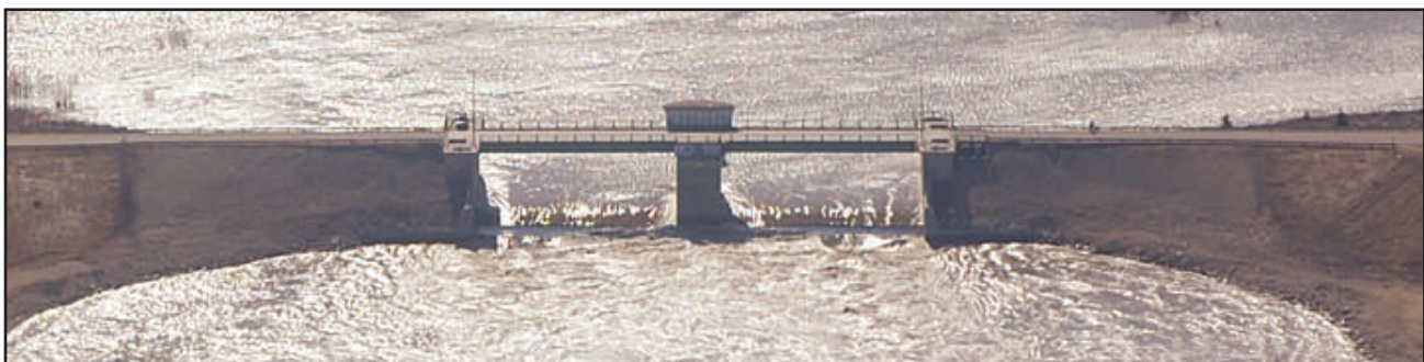
Figure 2-5: Inlet Control Structure viewed from downstream.
